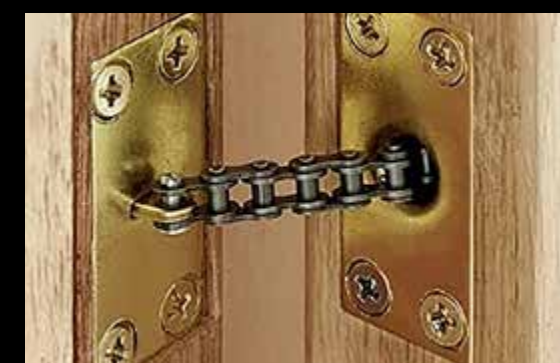
Example of an internal self-closing device
