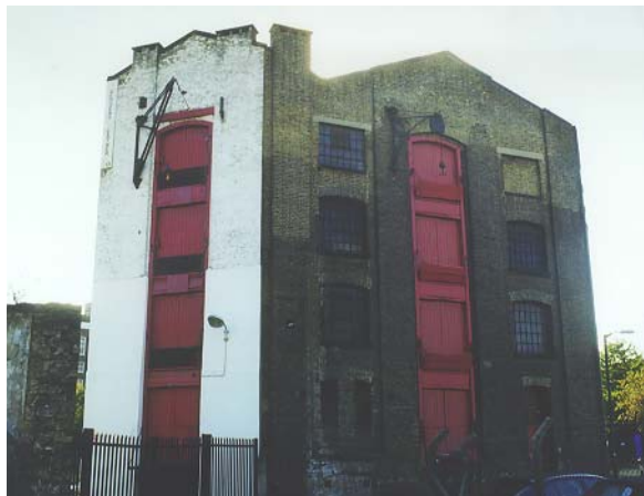
Figure 60 Vinegar Yard warehouse: any renovation should also consider the yards and spaces around it, which are currently used for car parking.
