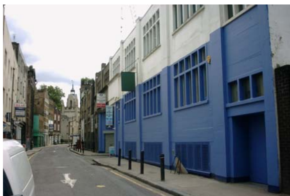
Figure 22 Looking south to St. Mary Magdalene, showing concrete buildings at 156-170 Bermondsey Street, with repaired and painted façades.
