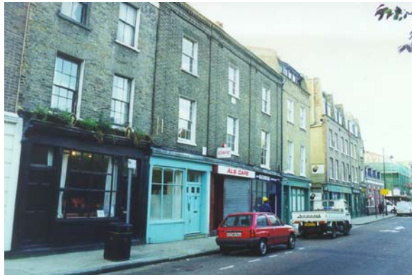
Figure 21 124-132 Bermondsey Street: early 19 th century houses converted to shops and now listed. The picture shows the importance of the original cornice line and the impact of modest roof extensions on neighbouring buildings.
