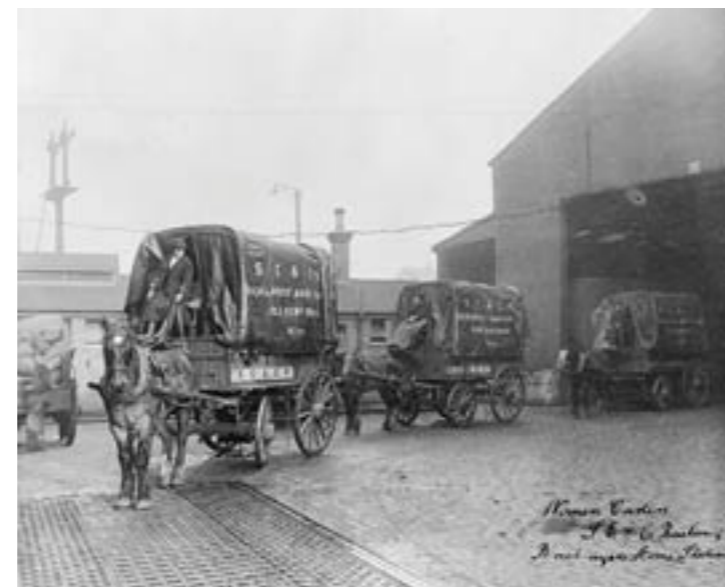
Figure 19: Bricklayers Arms' depot, 37 Old Kent Road.
