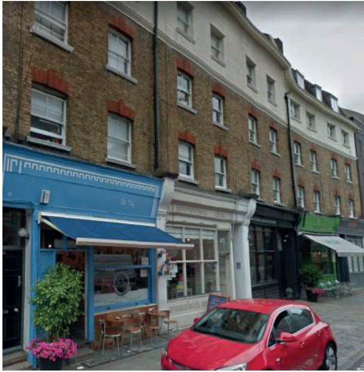
Parade of Shops, Snowsfields - north of the line of segregation proposed in EiP 181A
