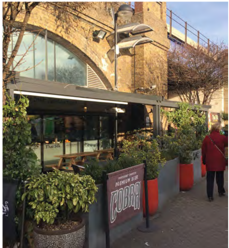
Railway Arches, Bermondsey Trading Estate
