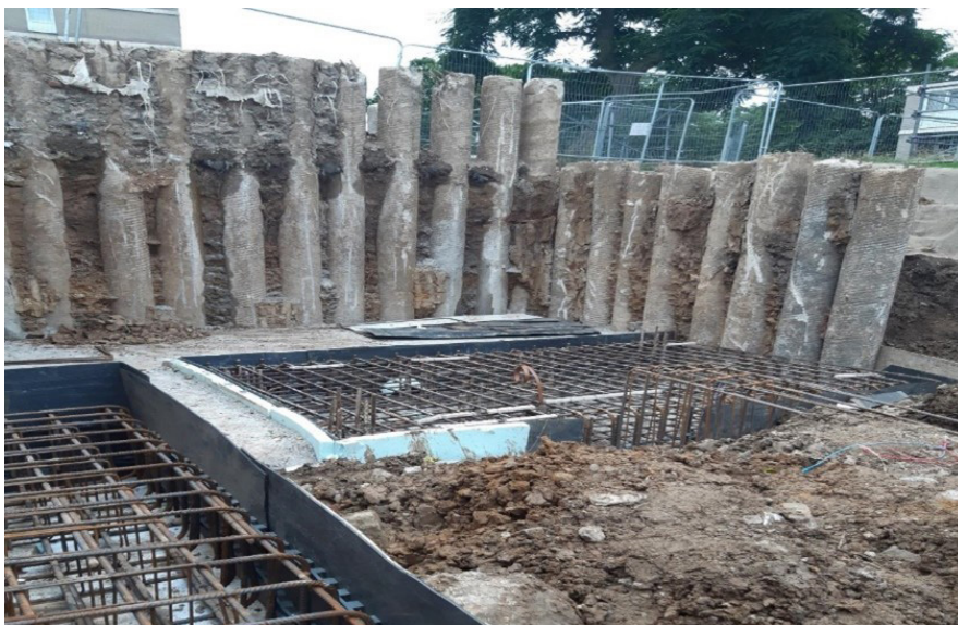
Steel reinforcements - Block B
