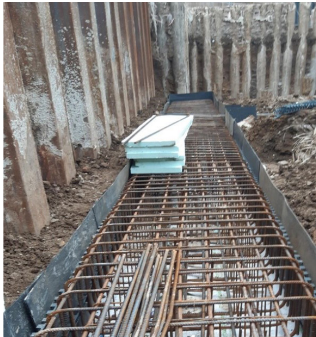
Steel reinforcements - Block B
