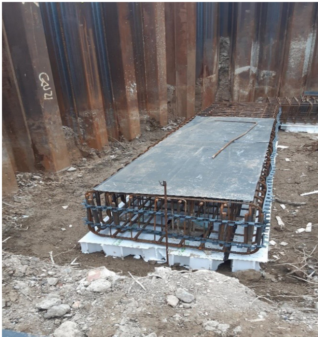
Steel reinforcements - Block B
