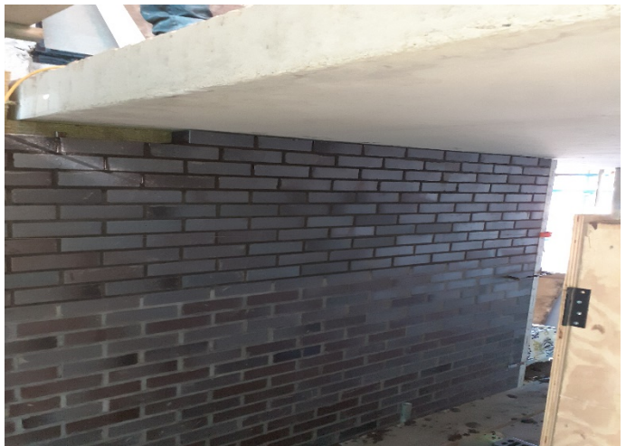
The communal landing area outside the lift
