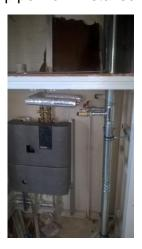
We can confirm that if the HIU is not connected, the valves shown on the attached photograph will be permanently capped off (they are currently capped off and are uncapped for the HIU installation only). Even if you open the valve, there will be no water.
