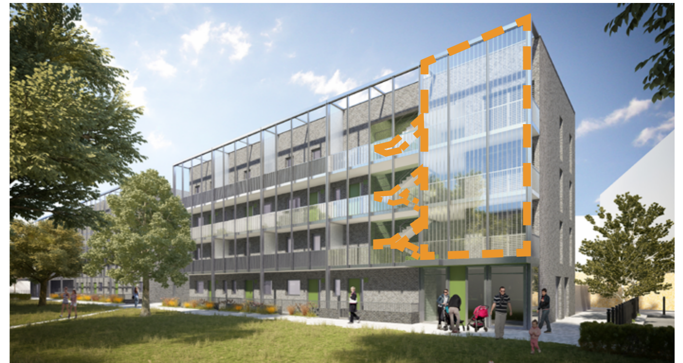
The visual above illustrates where the Racine access stair was previously located towards the front of the block. This has now been enclosed as indicated in plan (left). The glazed aspect has also been omitted.
