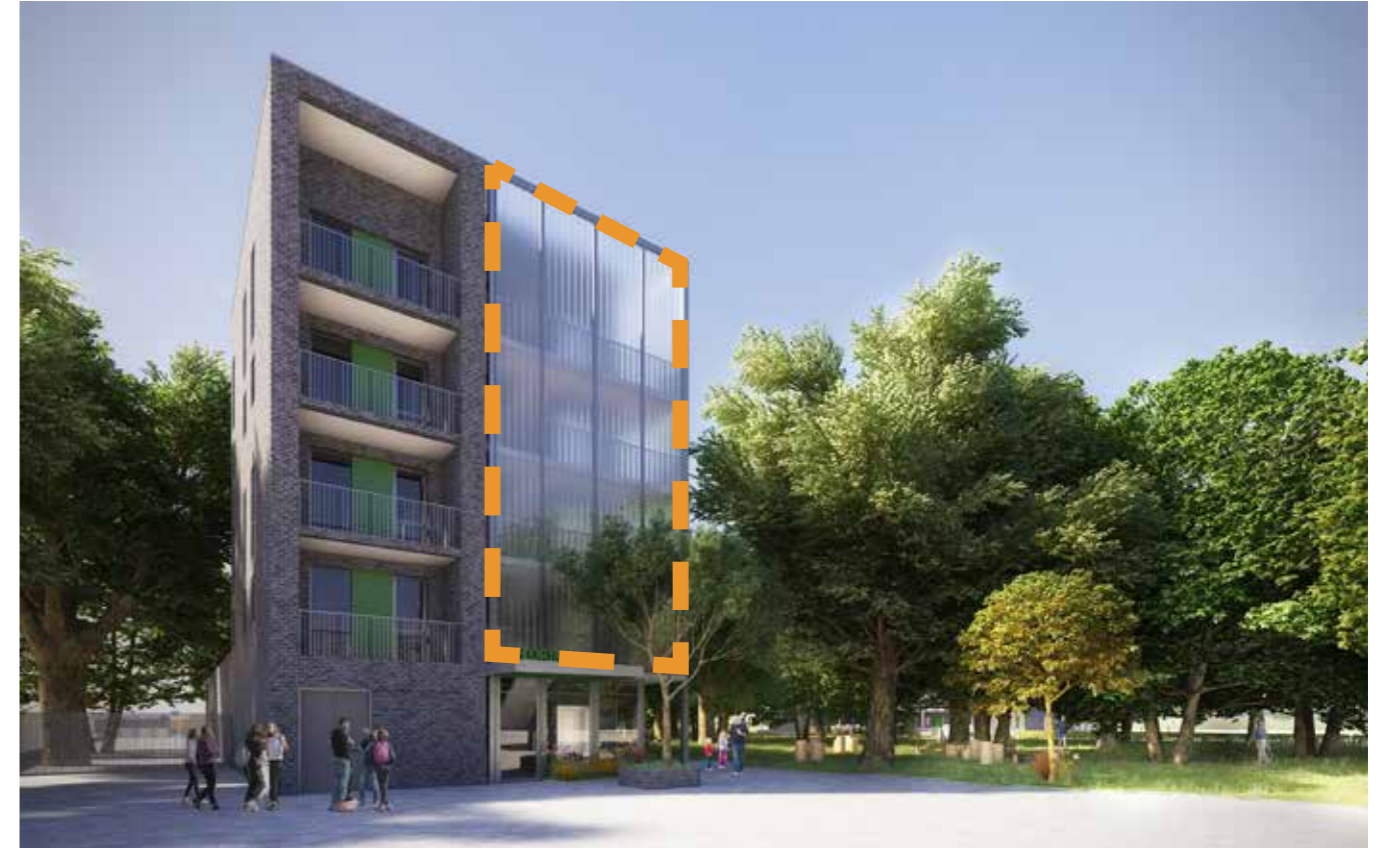
The visual above shows a glazed screen to the end facade of the Florian block, which was providing cover to the external stair. As the stairs are now enclosed this glazed aspect has been omitted.
