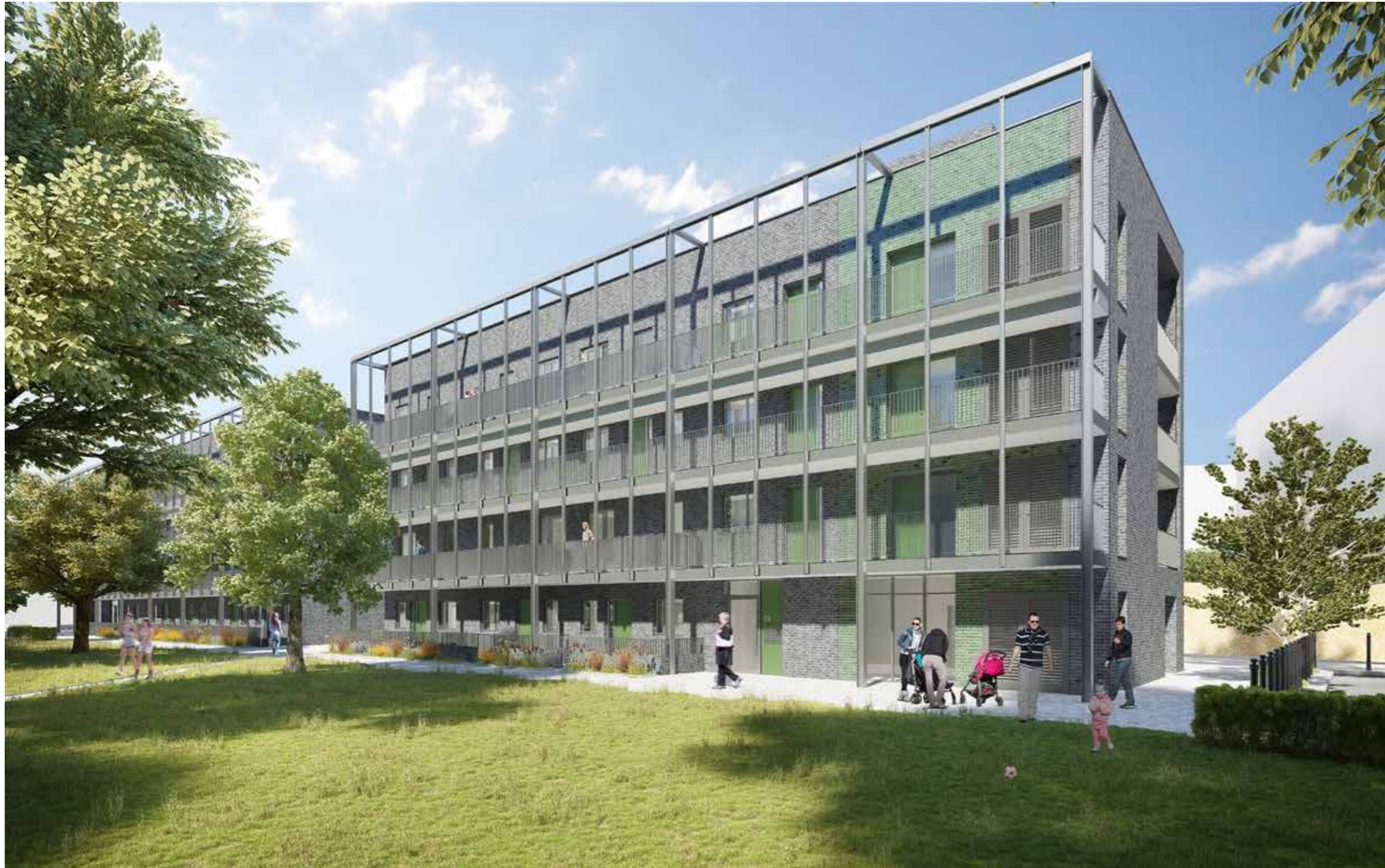
Racine North elevation facing onto central gardens
