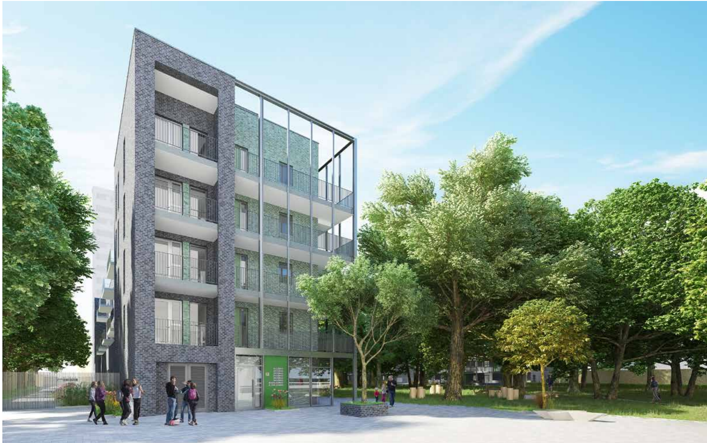
Florian South side elevation facing onto entrance square next to Florian Shops proposal
