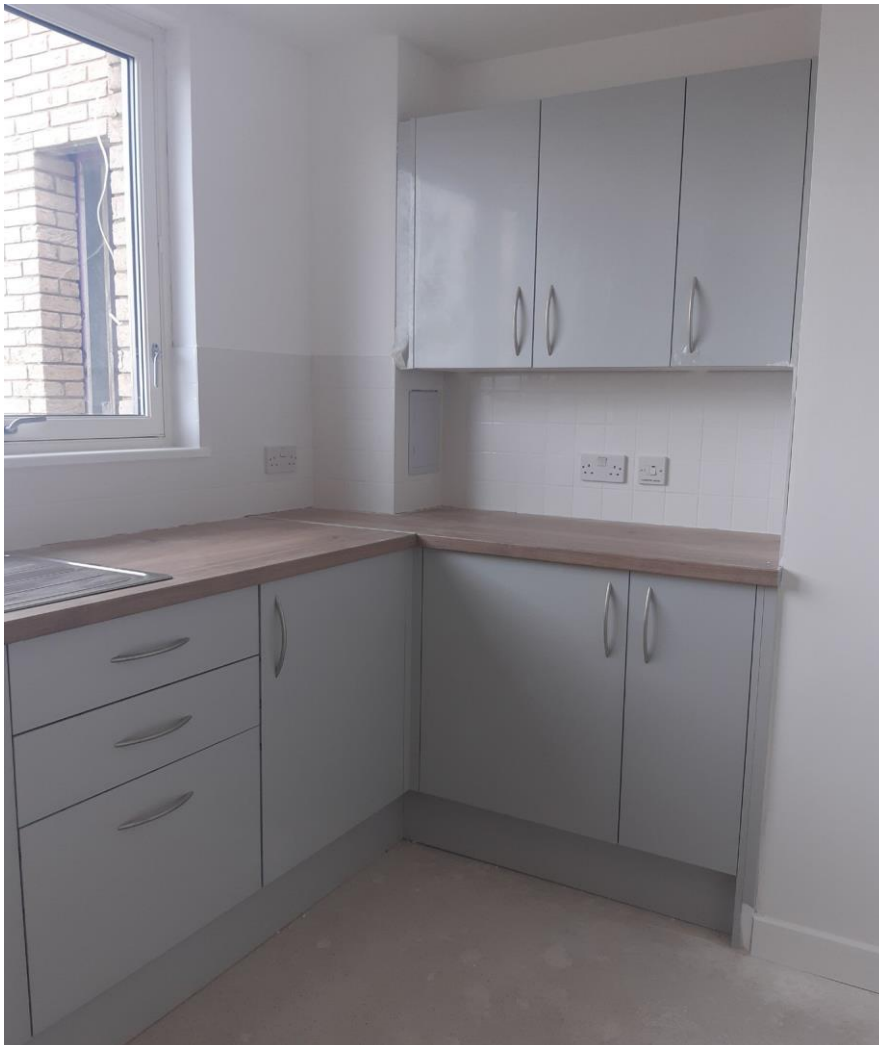
New kitchen installation near completion
