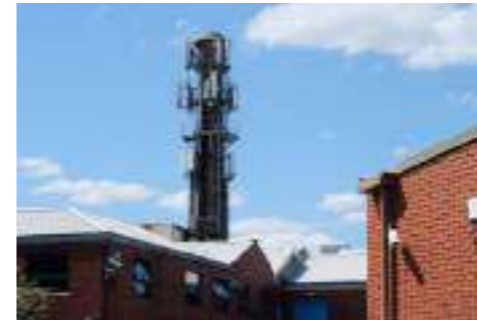
1 Historic brick chimney to remain visible landmark at the centre of the site
