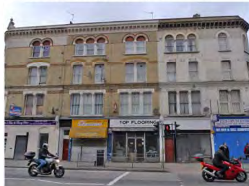
Photo 55: Nos. 36-44 Walworth Road
