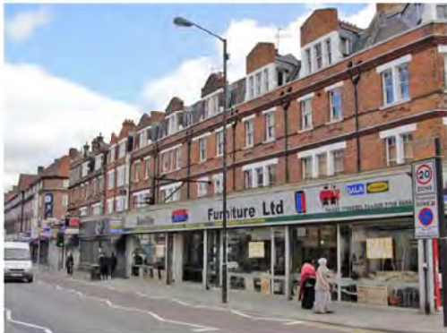
Photo 54: Nos. 49-67 Walworth Road
