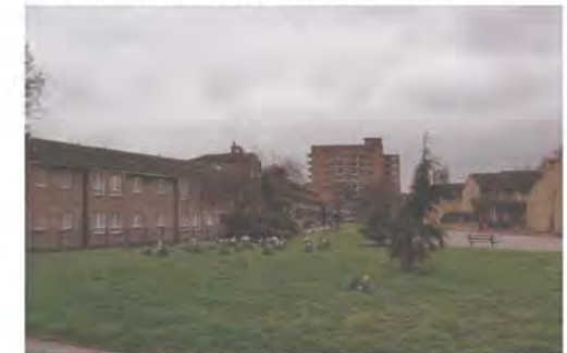
Canterbury Place, Newington Estate: this 'green corridor' should be improved where possible
