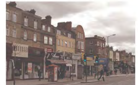
East side of Walworth Road: quality and cohesiveness of shop fronts should be addressed
