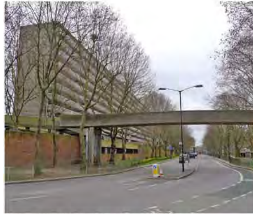
Photo 14: High level walkways of Heygate Estate
