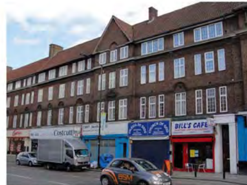
Photo 52: Camgate Mansions, Walworth Road
