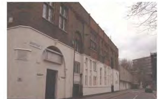
Corner of Thomas Doyle Street and Rotary Street: Opportunity to refurbish historic buildings
