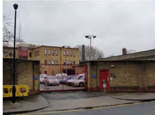
Photo 23: Amelia Street, rear of Police Station
