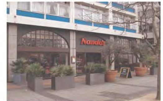
Base of Metro Central Heights: encourage active uses at ground floor level
