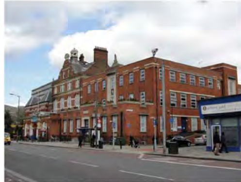
Photo 51: Civic complex (grade II listed), Walworth Road
