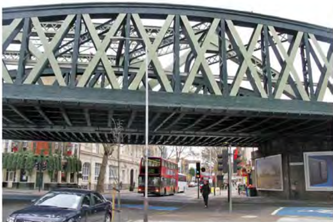
Photo 29: Victorian rail bridge, Borough Road
