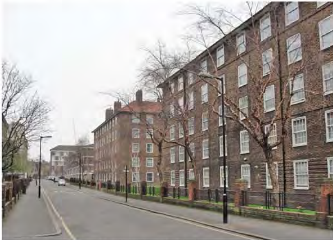
Photo 40: Banks House and Brunlees House, Bath Terrace
