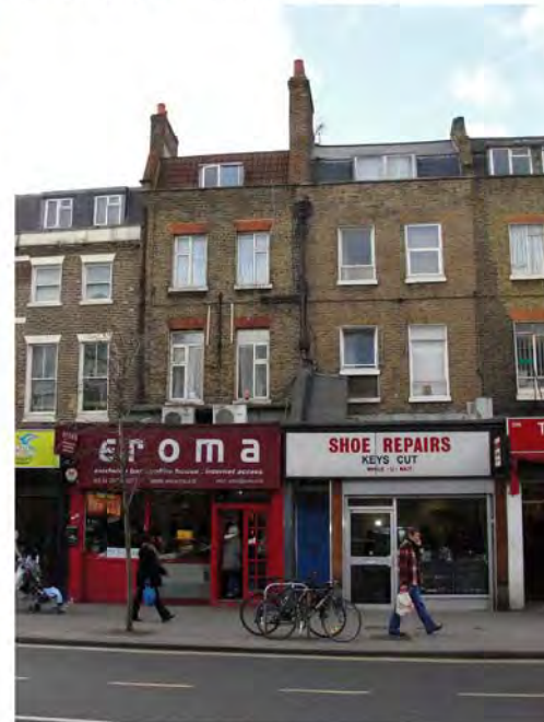
Photo 56: Nos. 294-298 Walworth Road
