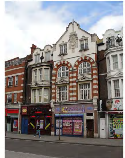
Photo 57: Nos. 353-357 Walworth Road
