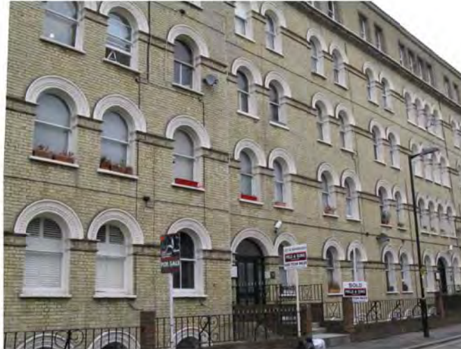
Photo 39: Devonshire, Bath and Trinity House, Bath Terrace
