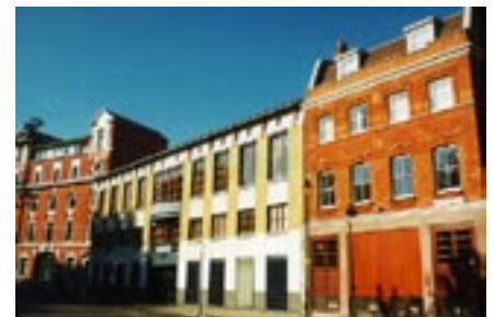
Figure 7 Modern development slotting effectively between Victorian buildings around Dockhead
