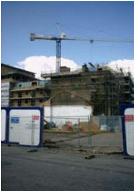
Figure 19 Warehouses at east end of Conservation Area are current undergoing redevelopment
