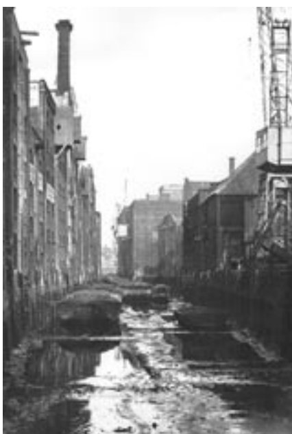
Figure 6 St Saviours Dock at low tide
