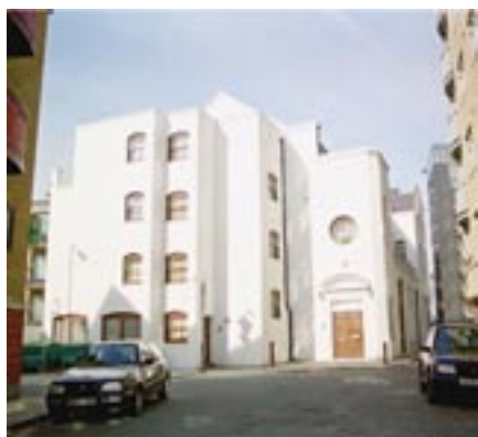
Figure 31 No 21 Bermondsey Wall West has recently been restored
