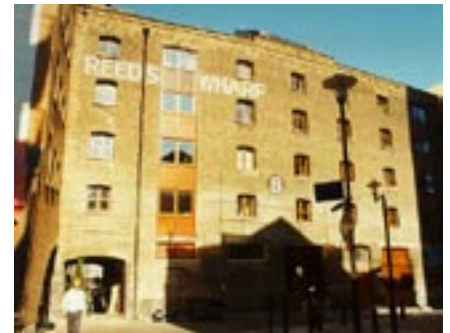
Figure 9 Reeds Wharf showing the typical features of a wharf building
