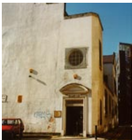
Figure 32 No 21 Bermondsey Wall West prior to restoration
