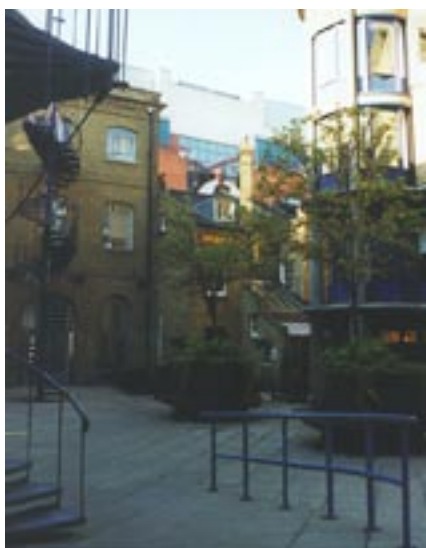
Figure 33 (middle and bottom) Tower Bridge Piazza is a successful civic spaces enlivened by a fountain and container planting – redevelopment enclosing the space follows the precedent of tall buildings.
