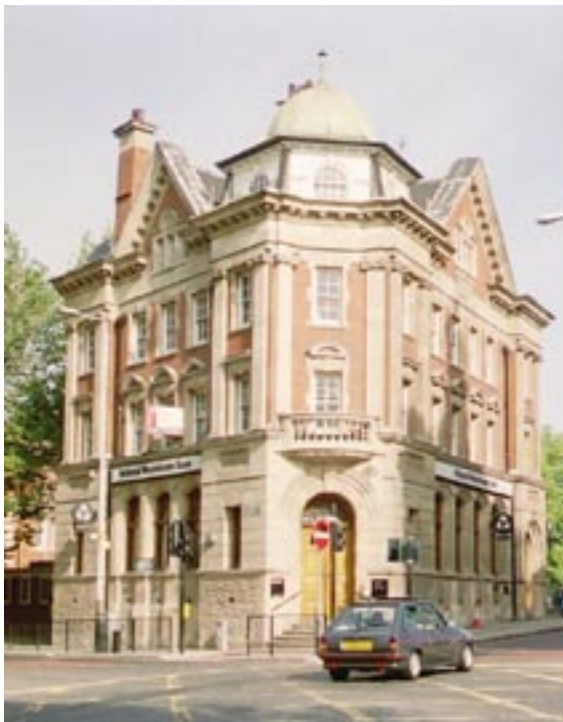
Figure 11 Buildings on Tooley Street have an elaborate civic style characteristic of the late 19th century. The former London & Counties Bank, 185 Tooley Street.
