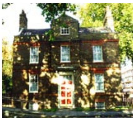
Figure 31 (right) The vicarage, no. 10 Fair Street.
