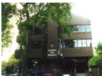
Figure 32 Nasmith House is built on the plinth of the 18th century St John Horselydown church.
