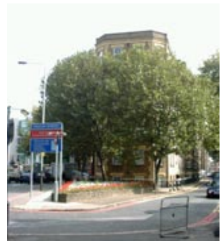
Figure 35 (right) Devon Mansions at the junction of Tooley Street, Fair Street and Queen Elizabeth Street.
