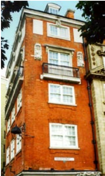
Figure 10 (left) No. 15 Tooley Street for the Bennett Steamship Company (1908) with artificial stone ornamentation.
