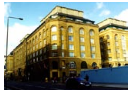
Figure 8 (right) The Counting House and Hay's Galleria from Tooley Street.
