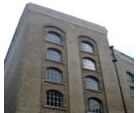
Figure 9 (left) The plain simplicity of the London Bridge Hospital and typical warehouse detailing.
