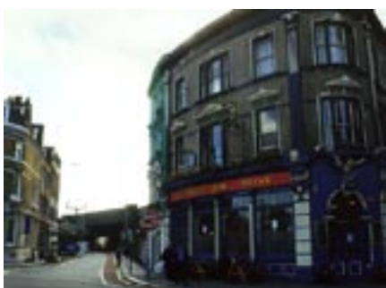
Figure 29 (right) Shipwright's Arms at the junction of Bermondsey Street
