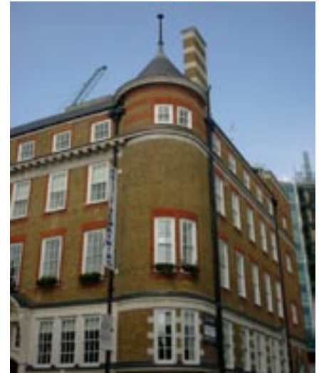
Figure 48 The old fire station has recently been restored to a high standard.
