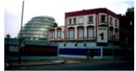
Figure 43 This former public house is one of the few remaining existing buildings on the north side of Tooley Street and forms part of an important group. The Greater London Assembly appears alien in this particular view, however, the More London Development will form a new backdrop to these buildings.
