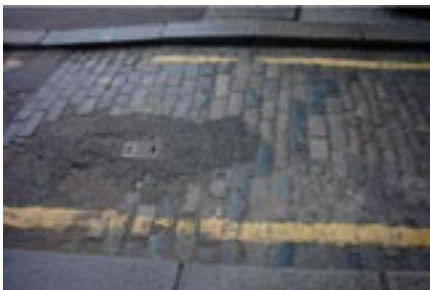
Figure 47 Where they exist, historic paving materials should always be properly reinstated (Shipwright Yard).
