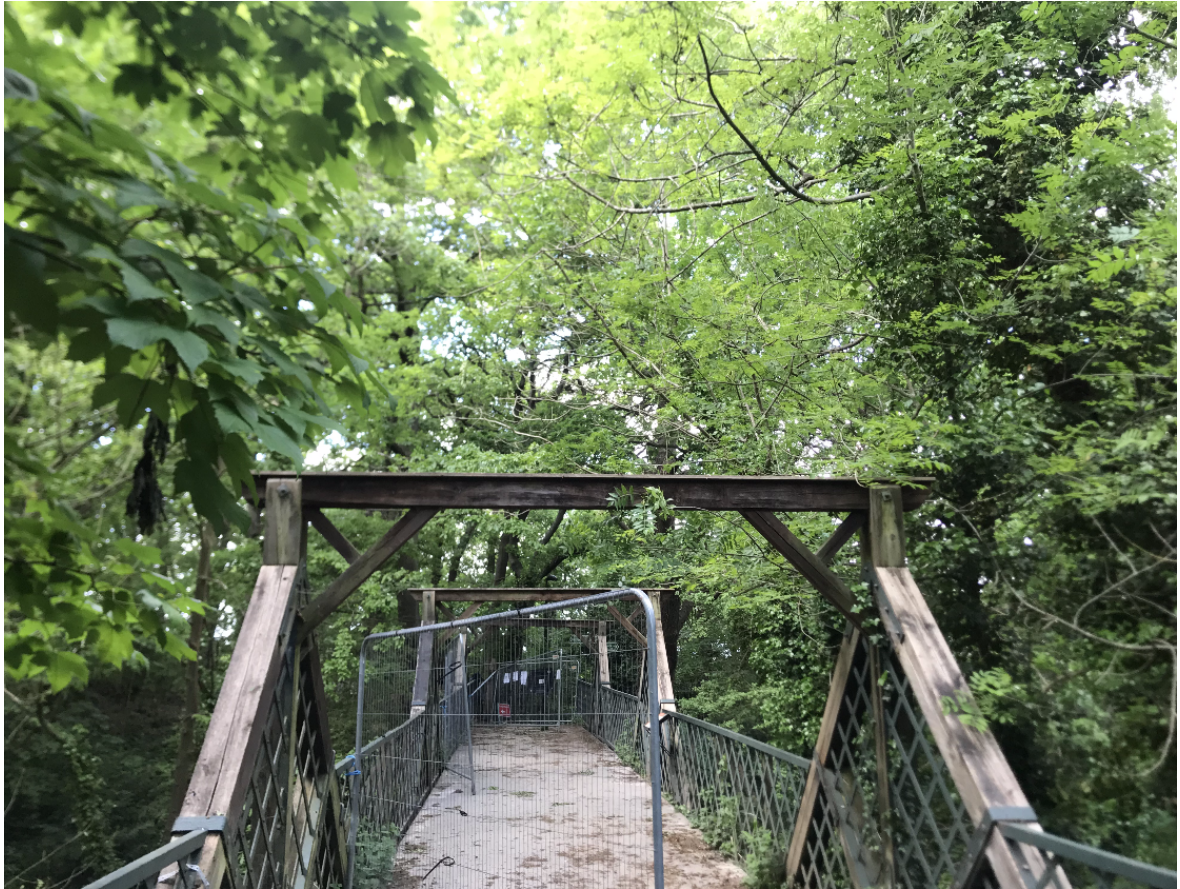
Photograph 1: Cox's Walk Footbridge
