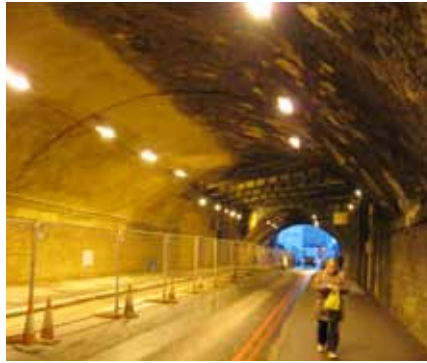
Bermondsey Street tunnel during the works
