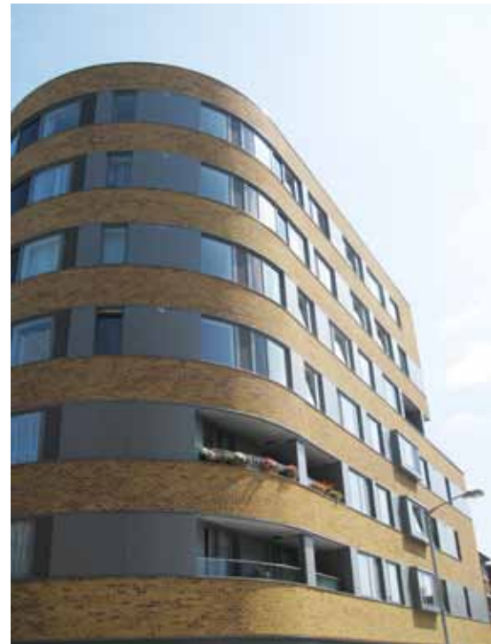
Affordable housing completed in Sweeny Crescent Bermondsey
