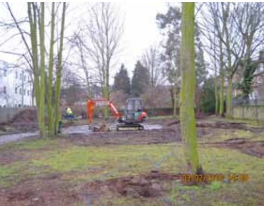
Mary Frobisher Park as works commence
