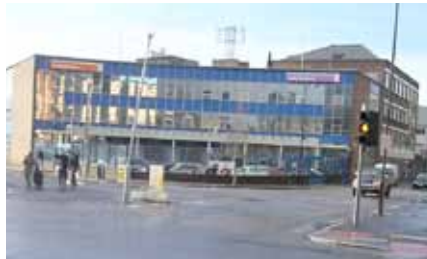
Great Suffolk Street junction with Webber Street before works
