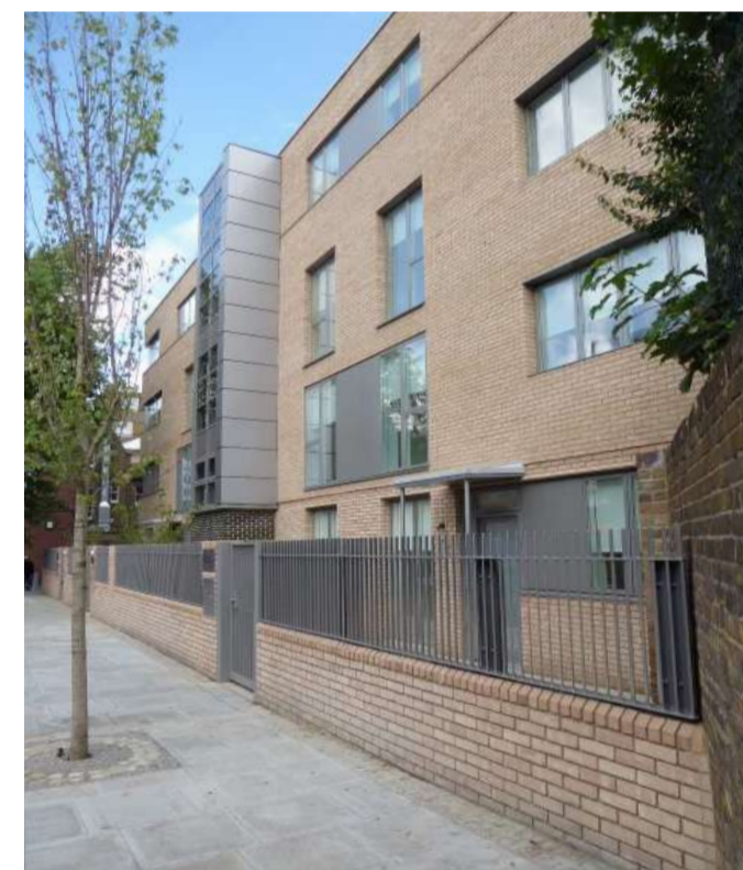
Clifton Estate / Clayton Road, SE5
