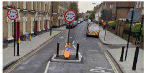
Width restriction island and signs to be removed
