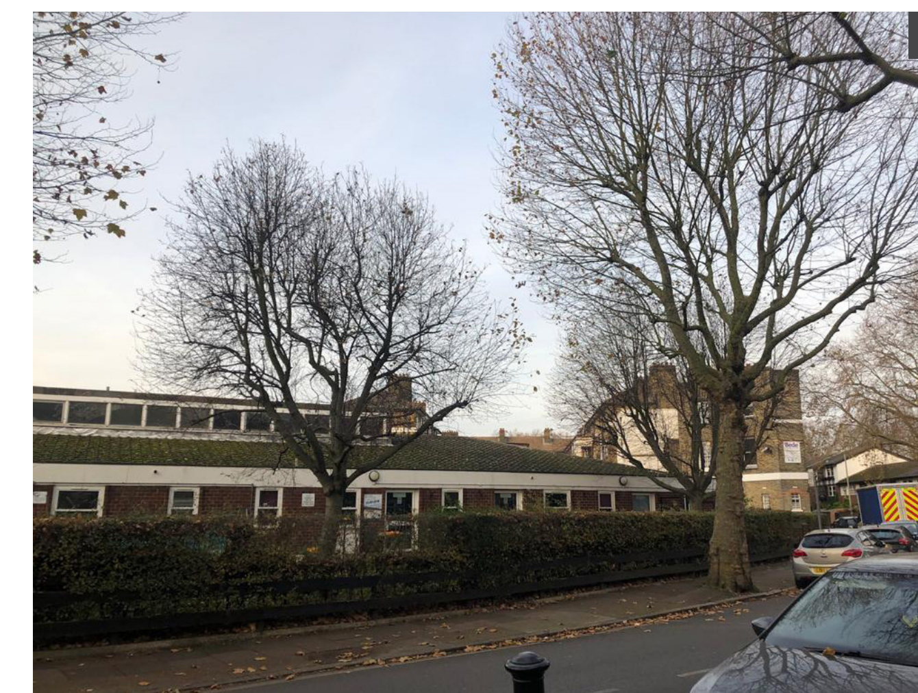
The disused Day Centre and mature trees
