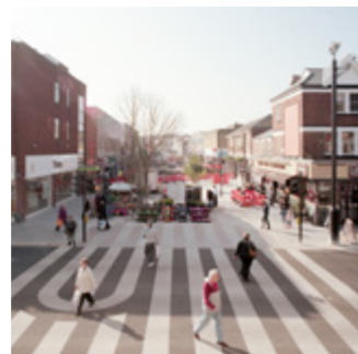
Material example: raised surface with paint treatment (East)
