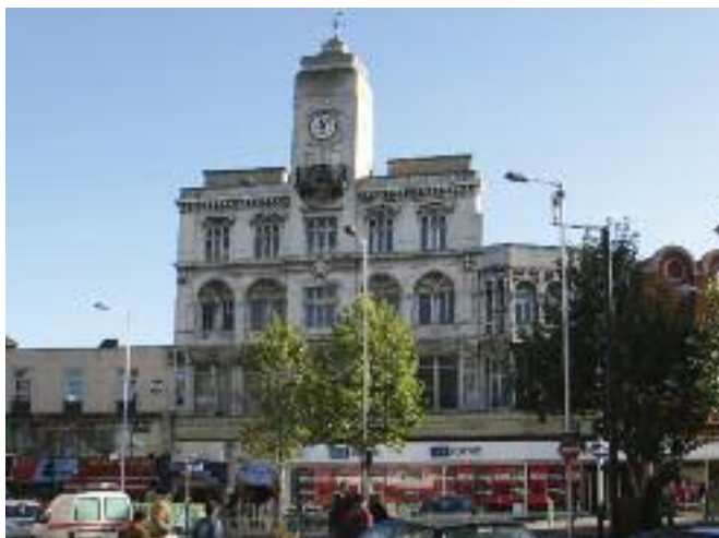
Former Jones Higgins department store building
