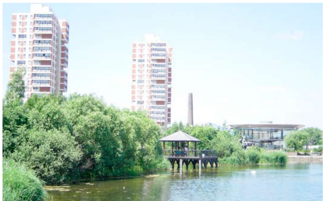
Canada Estate Towers
