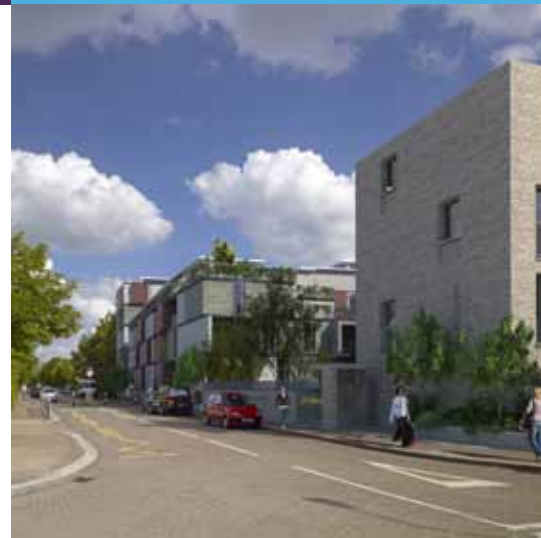
New housing on Mulberry Business Park
