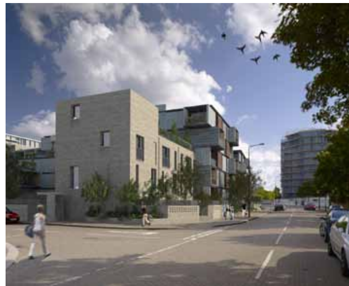
Four and five storey buildings on Mulberry Business Park
