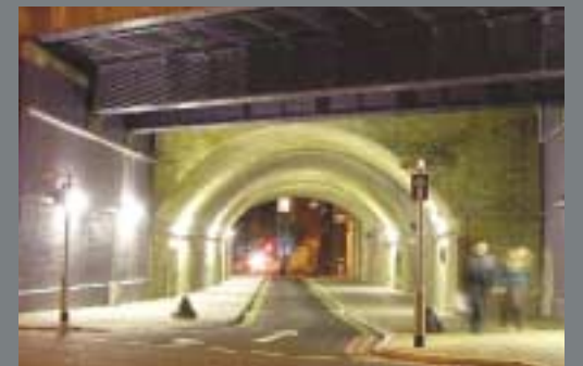
Refurbishment of the adjacent railway viaduct which has not only been cleaned, painted and given new lighting, but also has redesigned floorspace to create wider footways and a new cycle route.
