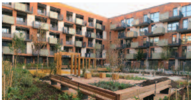
New homes at Manor Place
